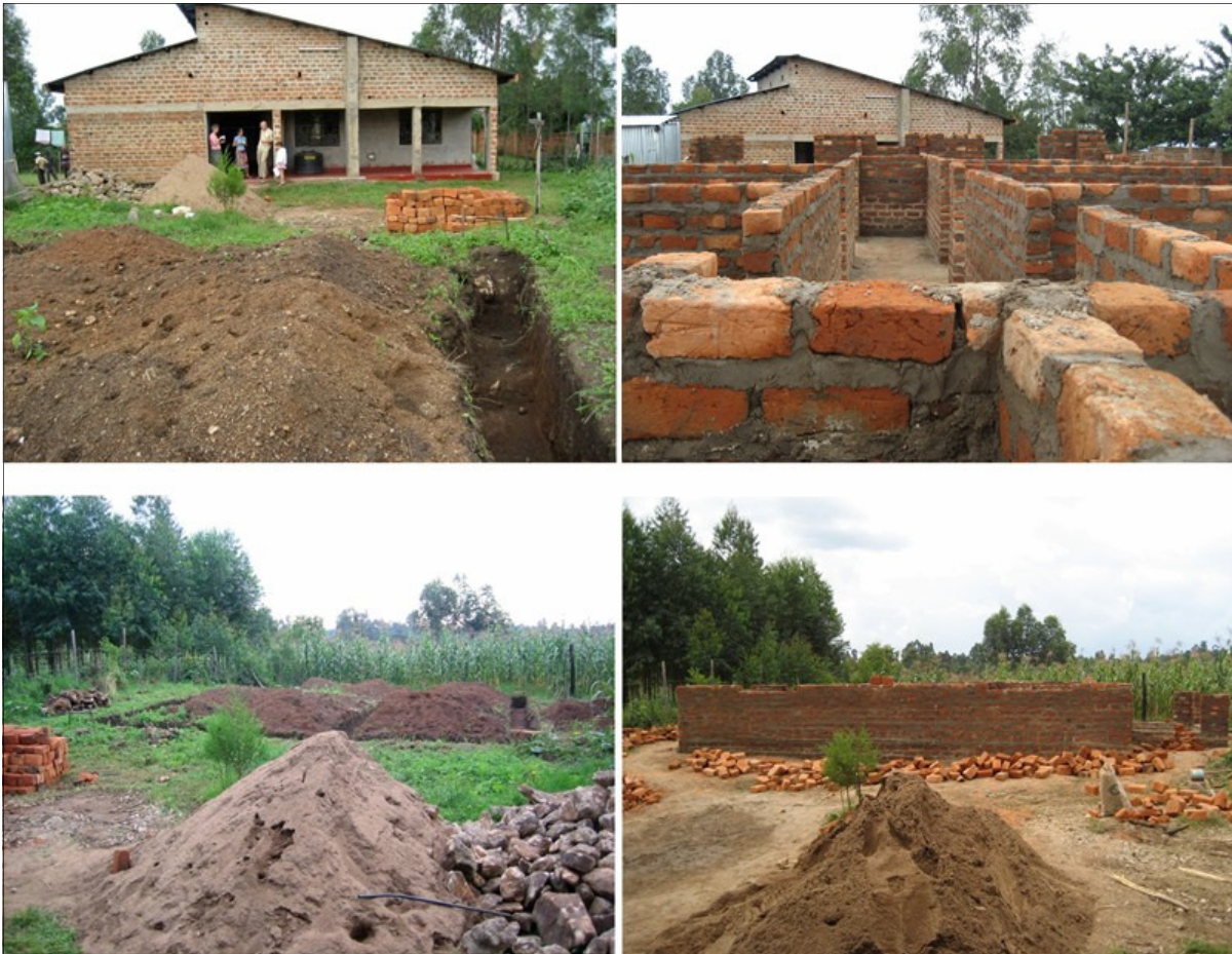
Before and after pictures of work done in Kenya.
