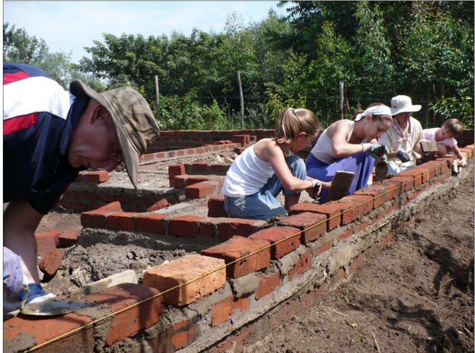
Building the walls of Friends Peace Center with willing hands.
