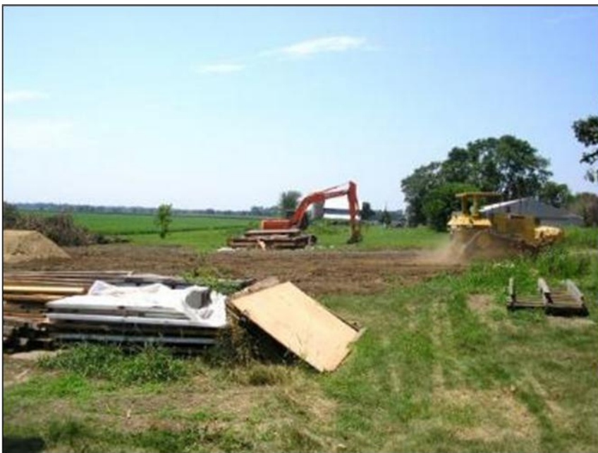
Ground being prepared for next phase of IYM vision
