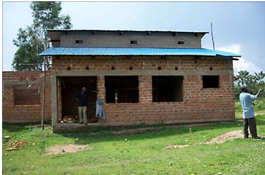
Work campers will continue building the Peace Center in Lubao, Kenya.
